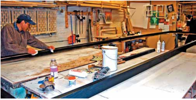
After the frame was joined, it received the final finish in the workshop.
